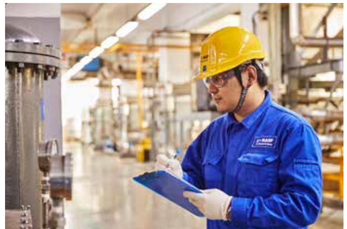
An operator inspects the pressure in the production facility.
