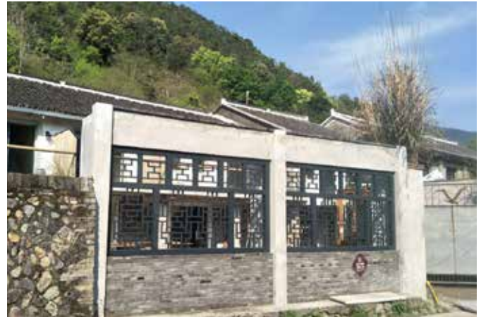
Using BASF's sustainable construction solutions, the granary will be transformed into a multi-purpose, efficient and modern guesthouse.
